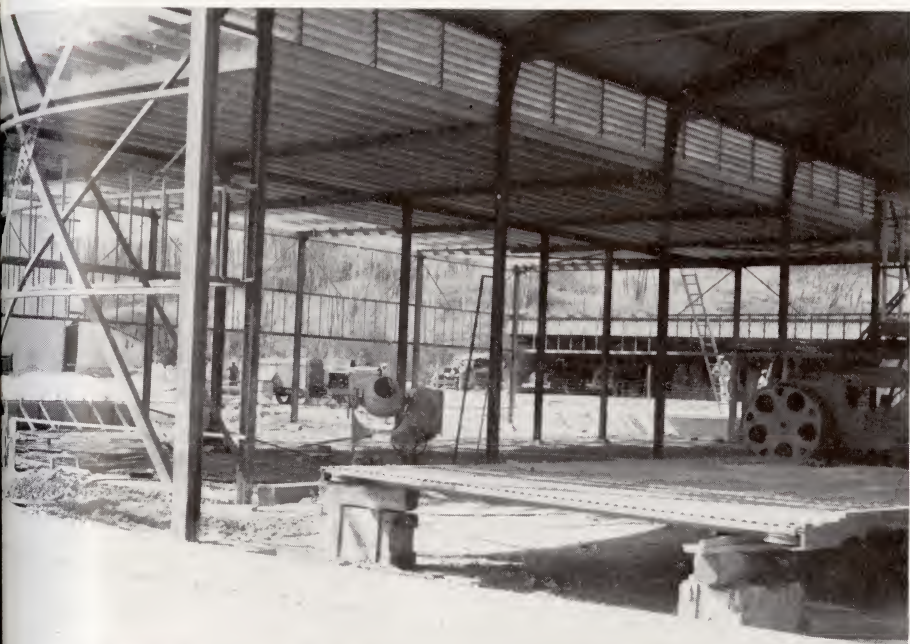
Workshops in construction, February 1940
